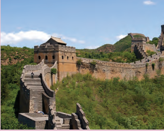
The Great Wall of China
